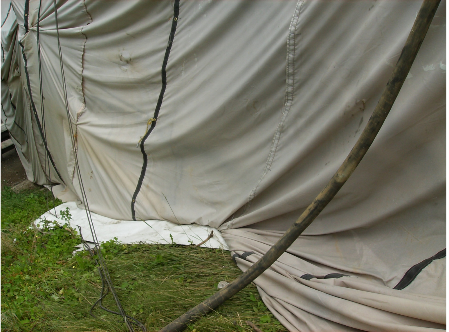
Side Containment Enclosure At Base
