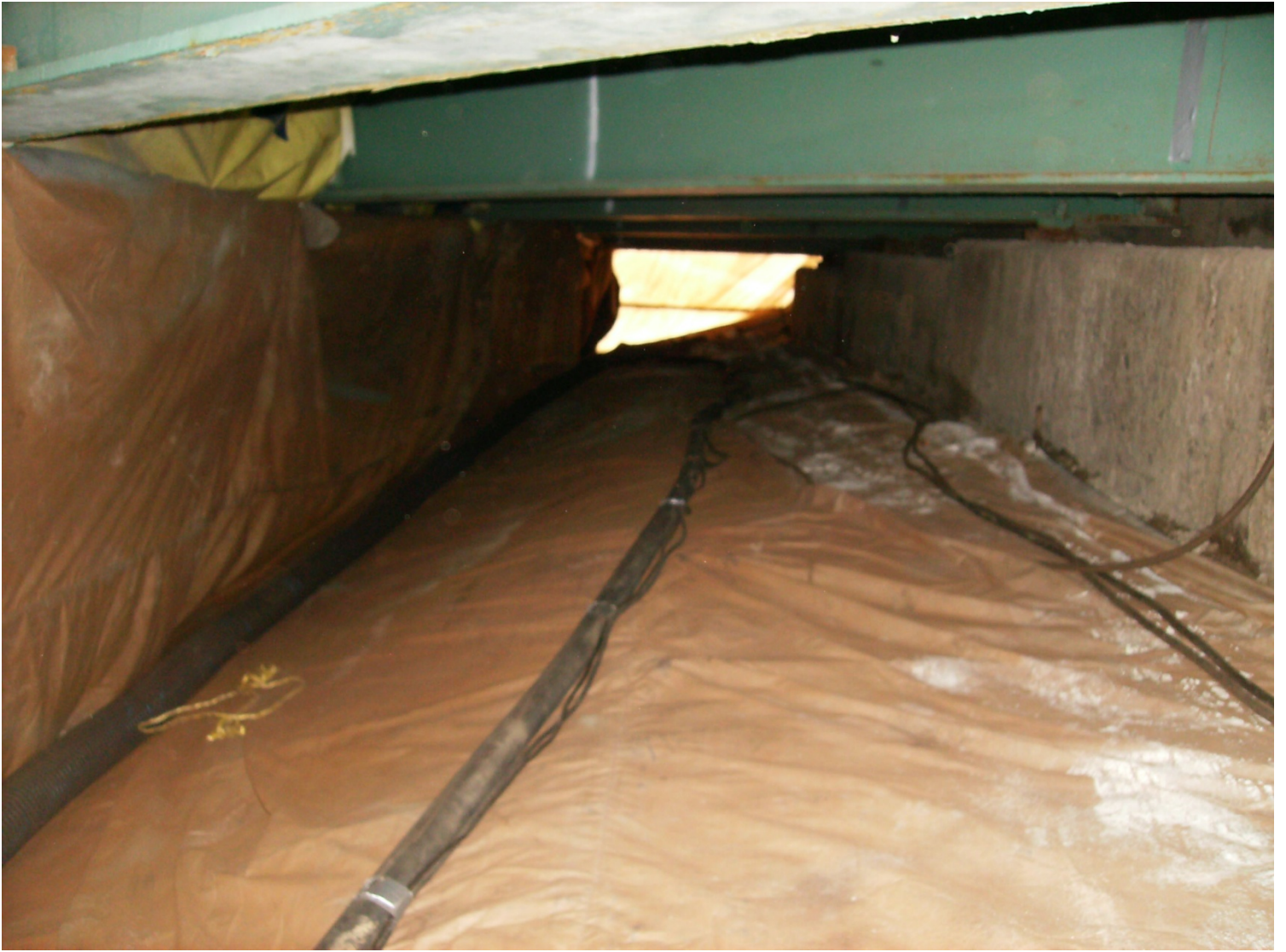
Containment System At Abutment
