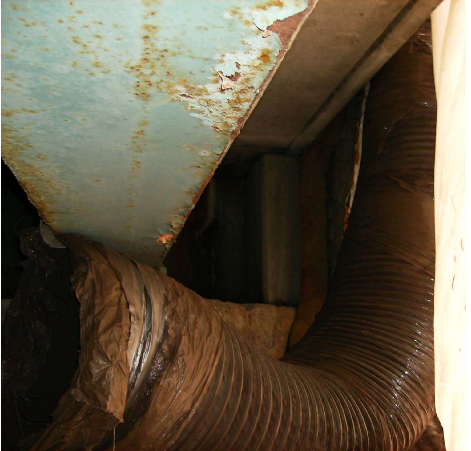
Dust Collector Hoses
