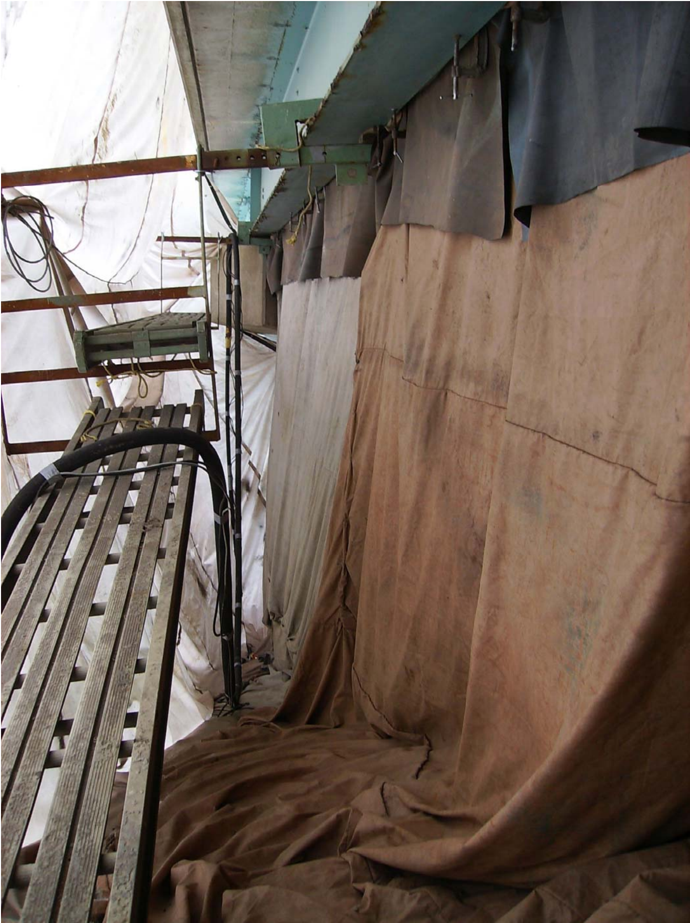
Containment System Interior w/Staging
