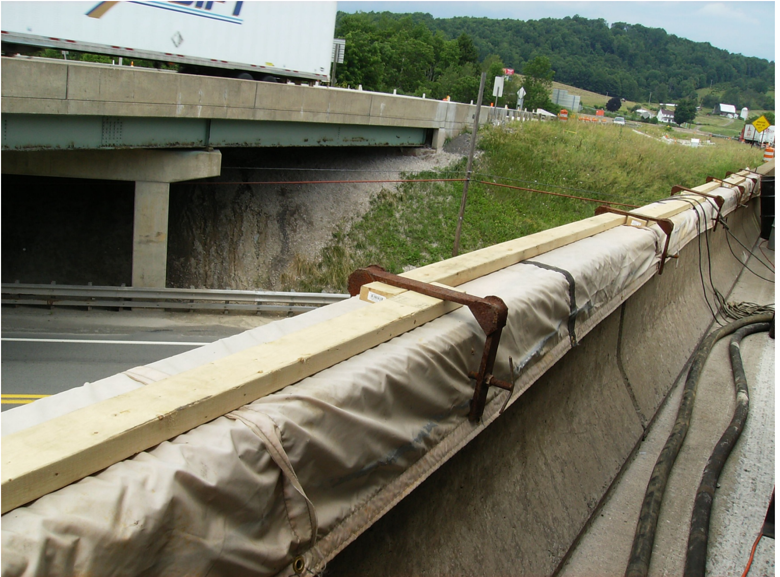
Upper Containment Attached To Concrete Barrier
