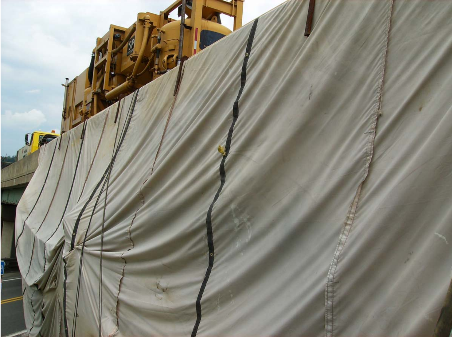
Side Containment Enclosure
